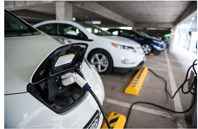
NREL Parking Garage – 108 Level 2 charging ports
